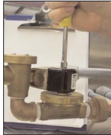
Removing the top screw
