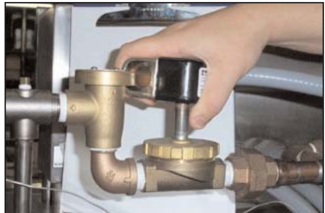
Removing the coil
