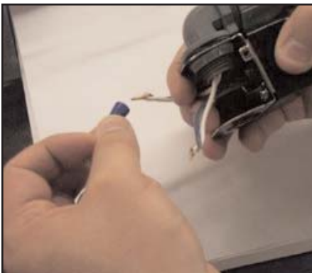
Removing the wire nuts
