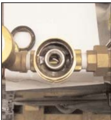
View inside the solenoid valve body
