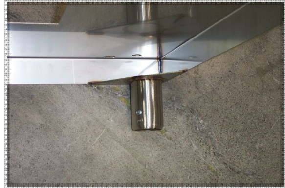
Figure 1—Leg socket showing set screw
