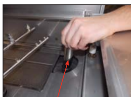
Removing the Standpipe
