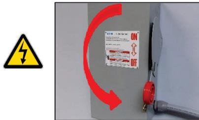
2. Confirm that the dishmachine is isolated from the power supply by attempting to power on the unit.
