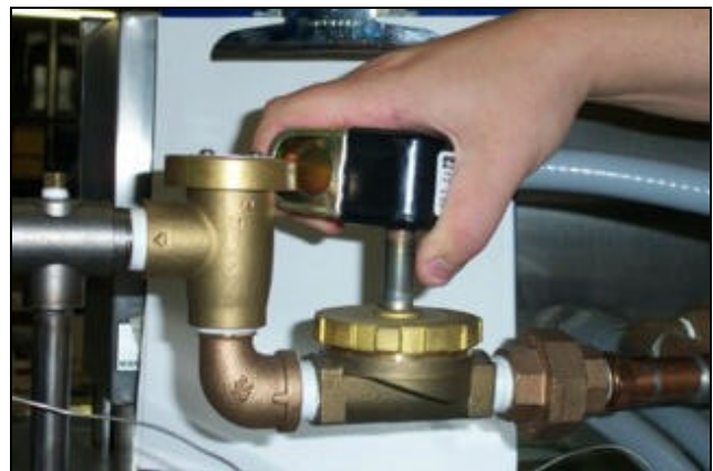
Removing the coil
