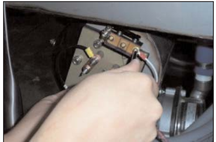
Securing jumpers to the thermostat.
