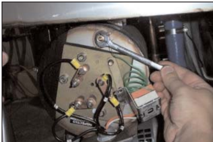
Removing the imperial brass fitting.
