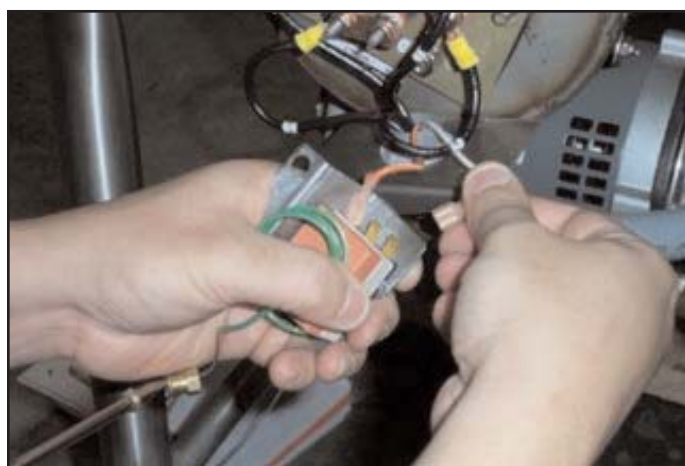
Removing the wires from the thermostat.
