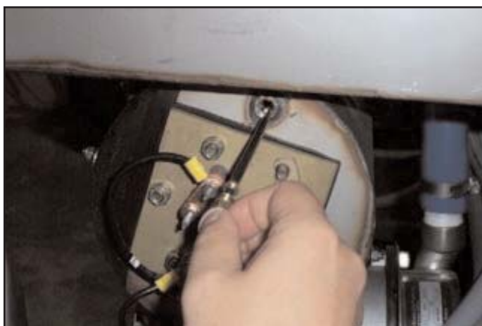
Pulling the thermostat probe and fitting from the well.
