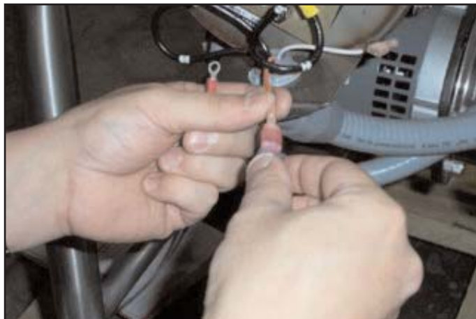
Attaching the jumper wires.
