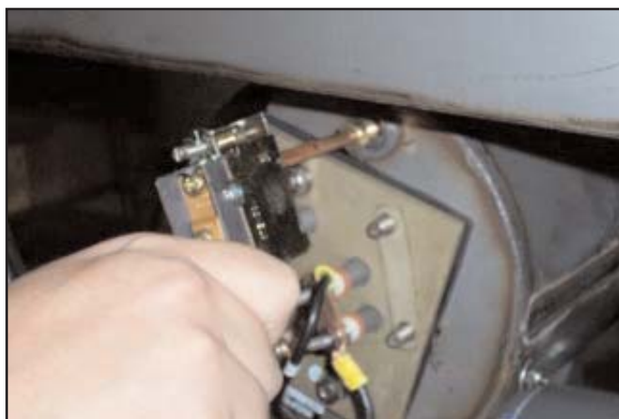
Putting the new thermostat in the well.
