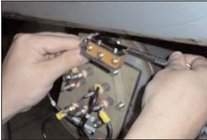
Tightening the brass fitting.
