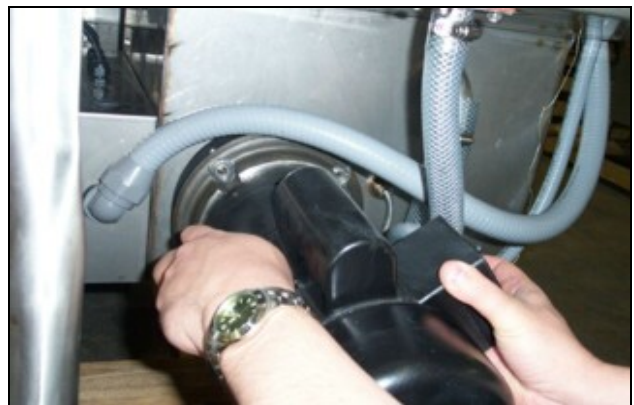
Remounting the wash motor assembly
