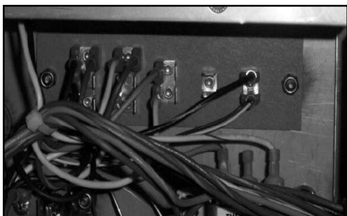
Terminal board inside the heater box
