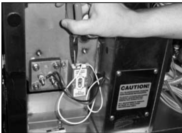
Removing the terminals.
