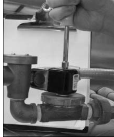
Removing the top screw
