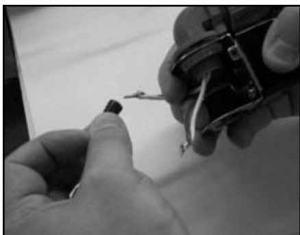
Removing the wire nuts
