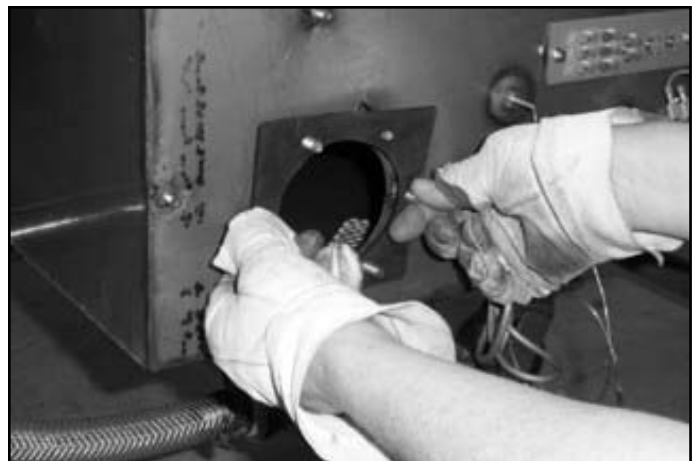
Removing the gasket
