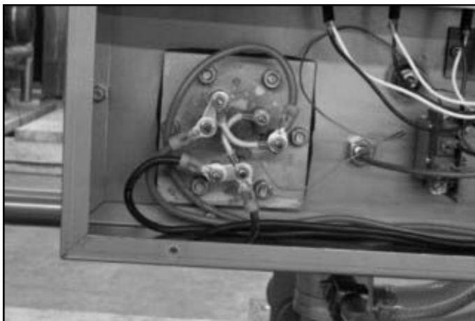
Single phase wiring
