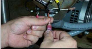
Attaching the jumper wires.
