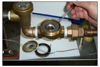
Removing the mesh strainer screen
