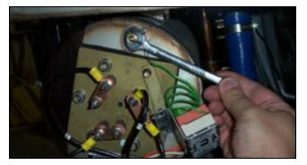
Removing the imperial brass fitting (Tempstar).
