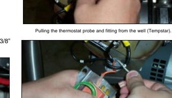
Removing the wires from the thermostat.
