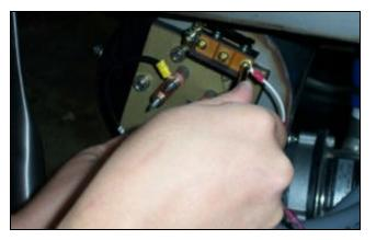
Securing jumpers to the thermostat.
