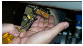
Removing the thermostat screws.
