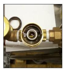
View inside the solenoid valve body
