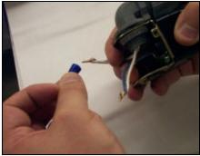
Removing the wire nuts
