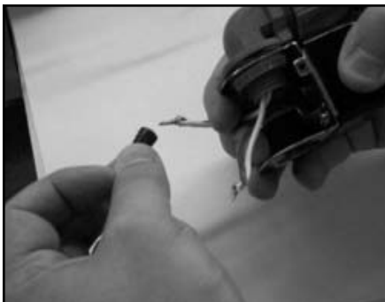
Removing the wire nuts
