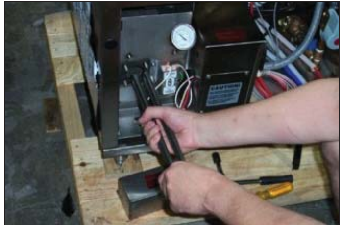
Pulling the heater out.
