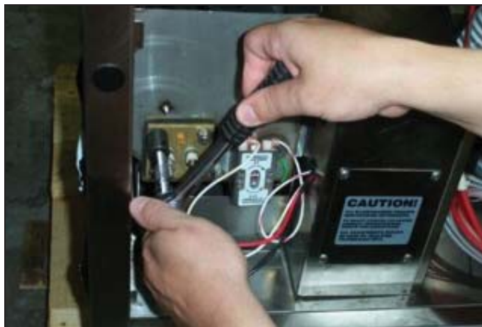
Using the ratchet to remove the heater mounting nuts.
