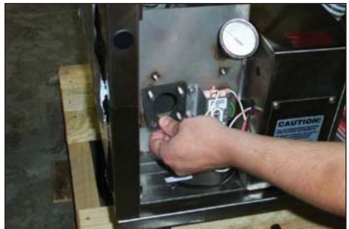
Removing the heater gasket
