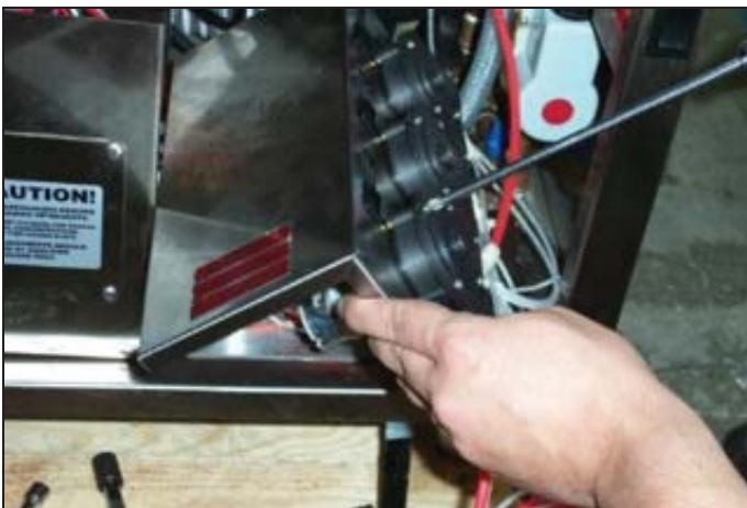
Removing the pump front cover screws.
