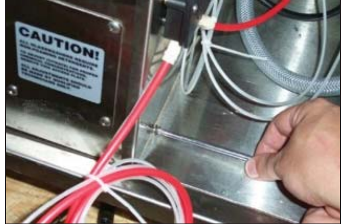
Removing the screws for the electrical box cover.
