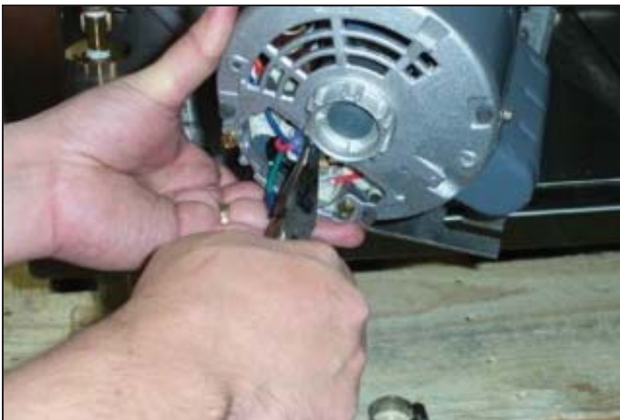
Removing the power wires.
