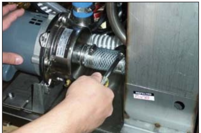
Loosening the suction hose clamps.
