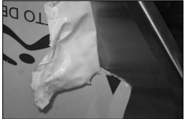
Remove any protective plastic prior to installation.
