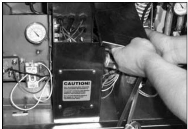
Removing the electrical box cover.
