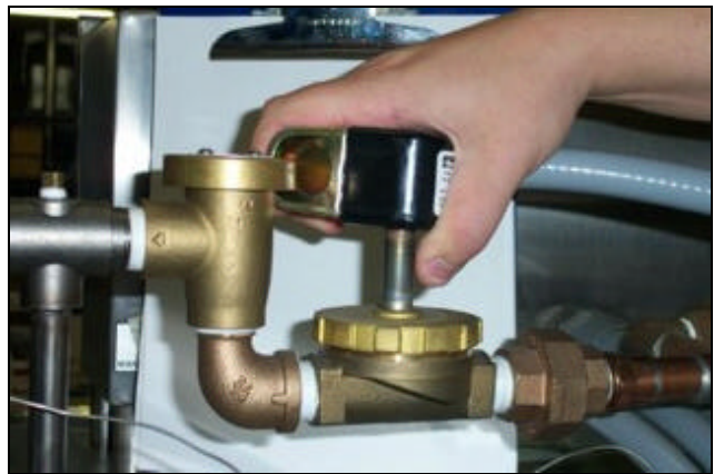
Removing the coil
