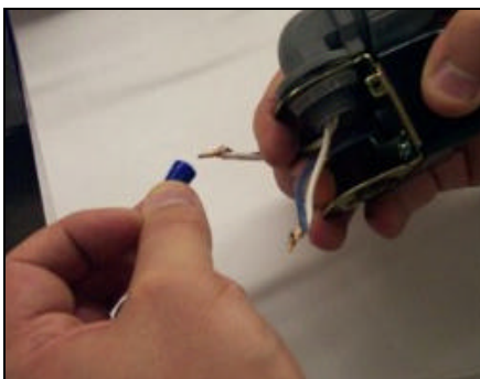
Removing the wire nuts
