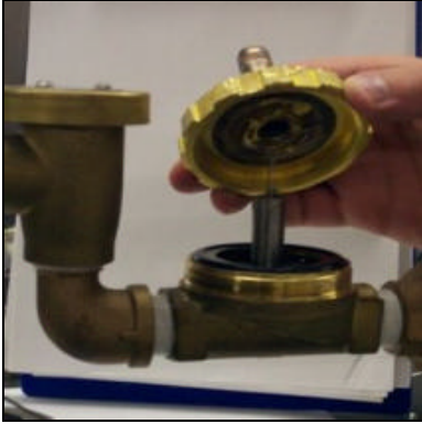
Removing the valve bonnet
