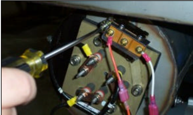
Calibrating the new thermostat.
