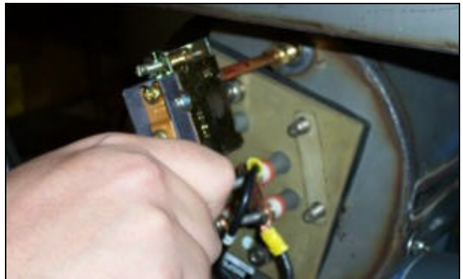
Putting the new thermostat in the well.
