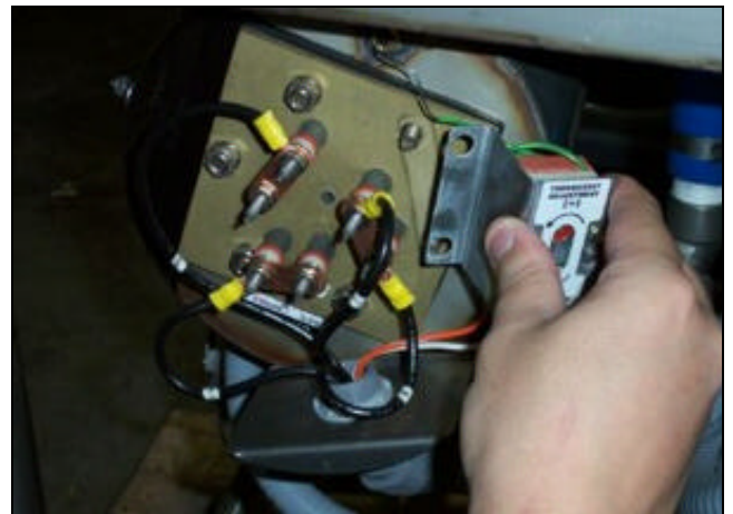
Removing the thermostat bracket.
