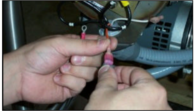
Attaching the jumper wires.
