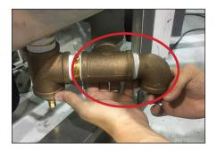
8. Remove solenoid coil from the 05700-004-14-95 assembly.
