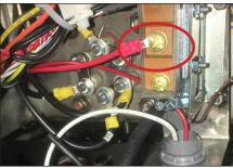
24. Connect the black wire from the SJ cord to the COMMON lug on the thermostat.
