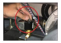
11. Connect the drain discharge piping (not supplied) to the Elbow, 04730-206-32-00, installed in Step 7.
