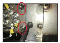
The thermostat can be turned either way depending on available space, etc. Just be sure to pay attention to which lugs are NORM OPEN, NORM CLOSED, and COMMON when connecting the wires in Steps 23 & 24.
