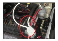
23. Connect the red wire from the solenoid coil to the NORM OPEN lug on the thermostat.
