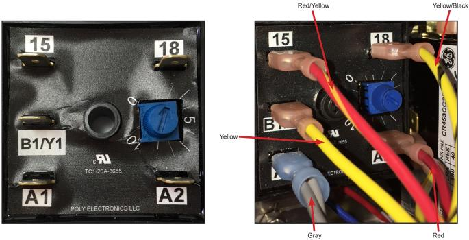
1. Using a flathead screwdriver, turn the blue knob until the arrow points at the "3" line.
