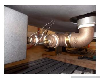
3. Connect user-supplied 115 V cord (from facility power) into solenoid box as shown below:
