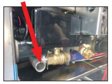
6. Using adjustable wrench, remove solenoid valve assembly.
