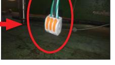
24. Disconnect red and white wires from machine 2-way gray/orange splicing connector and connect them to 3-way gray/orange splicing connector at end of red wire on Item #3 from kit.
