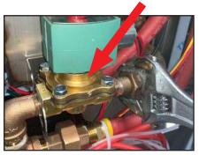
19. Re-install PRV removed in Step 8.
