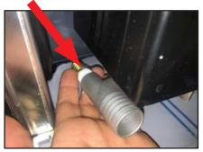
14. Put mini-clamp 04730-011-36-05, Item #7 from kit that shipped in the bag, on end of blue hose (orient clamp so it can be tightened later). Install hose onto barbed end of fitting installed in Step 12.
