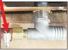
10. Using 1/4" nutdriver/socket or flathead screwdriver, tighten mini-clamp.
