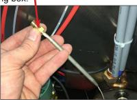
19. Insert the thermostat probe and fitting into the hole on the side of the drain water tempering tube.
