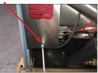
18. Place thermostat fitting from the kit on the thermostat probe attached to the drain water tempering box.
