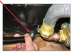
4. Put a clamp from the kit on the bottom of the 12" hose from the kit.
