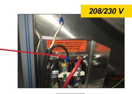
**NOTICE** After connecting and tightening, ensure black wire and incoming power wire cannot be pulled from the terminal block.
