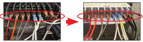
6. Disconnect orange wire and white wire connected to black wires on old timer.
